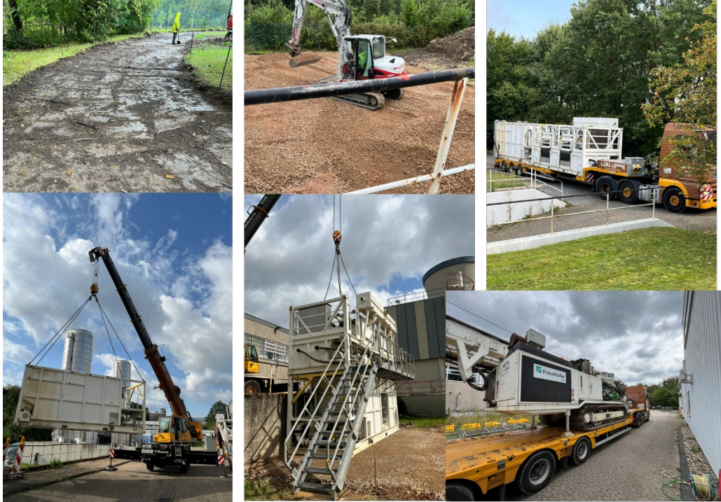
Figure 5: Construction of the demo site in Bochum
